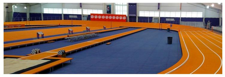
IN 1980, MONDO INSTALLED THE FIRST PERMANENT MODULTRACK BANKED TRACK AT THE PALAZZO A VELA IN TURIN. MODULTRACK PERMANENT TRACKS ARE FULLY COUPLED FOR EASE OF ASSEMBLY, TRANSPORTATION AND DIMENSIONAL ACCURACY OVER TIME. UNLIKE CONCRETE PERMANENT SOLUTIONS, THESE TRACKS CAN BE ASSEMBLED IN JUST A FEW DAYS, WITH NO NEED TO WAIT FOR THE FLOOR SCREED TO DRY.
