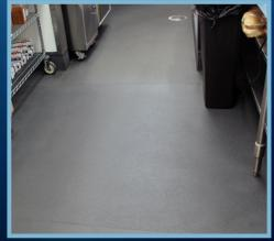
Aggressive floor surface texture provides the safest work environment for your staff. (coefficient of friction; dry 1.31 | wet 1.06)
